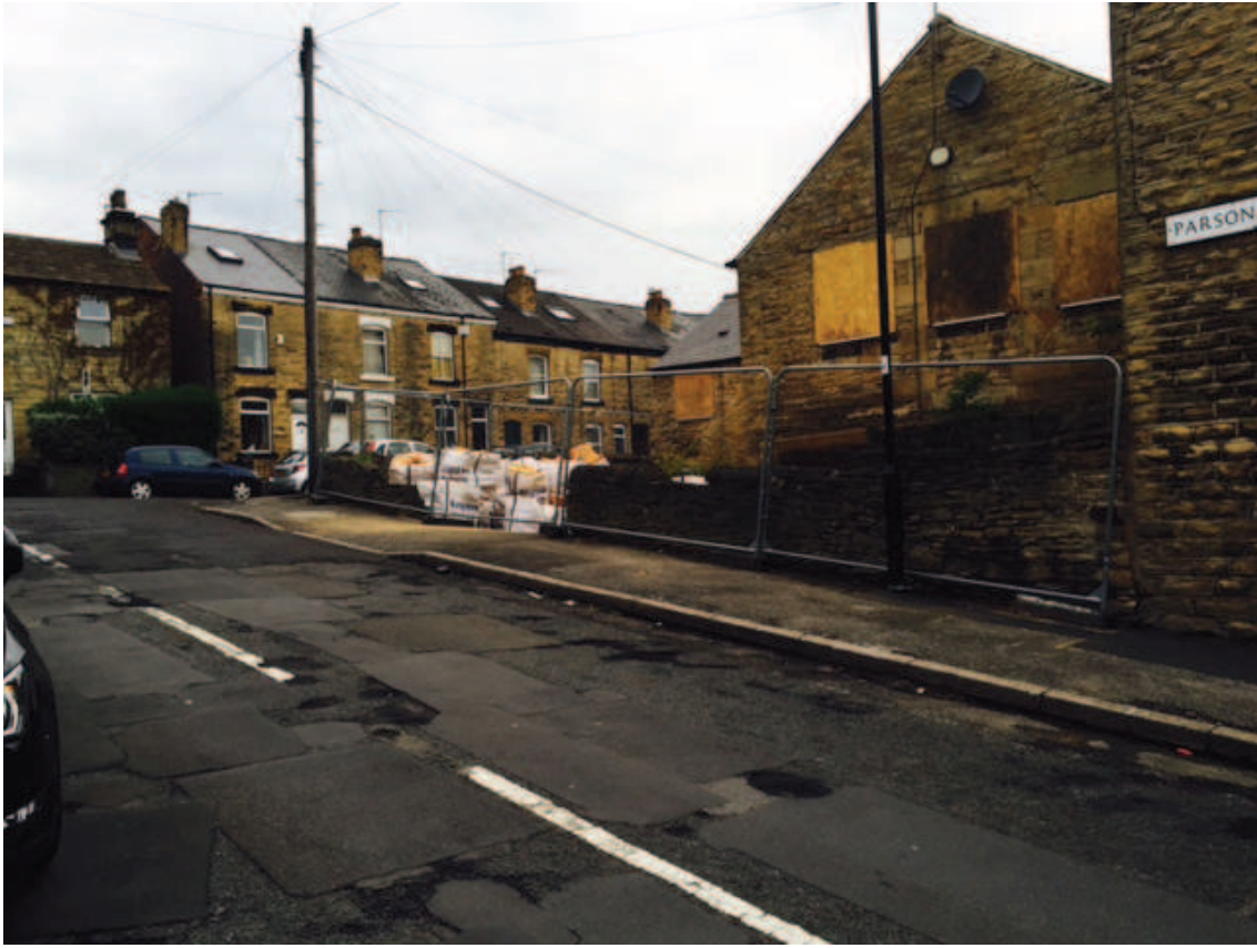
Figure 2 view of frontage of application site on Parsonage Street
